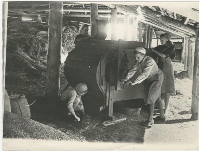
In the photo is a "Winnowing machine", a machine for cleaning the "pile" obtained by threshing. The heap consists, in addition to grain, of fragments of straw of different sizes, empty ears.
